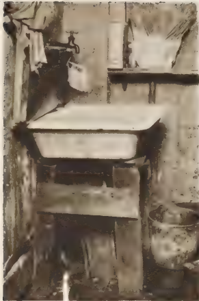
Right: A modernistic trend is shown in this compact washing nook, the creation of Crane Plumbing. The pail may be had in red for fire only.
